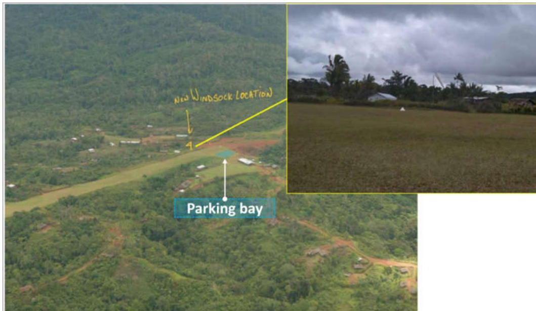
Figure 13. Dodomona Airstrip showing the newly installed windsock near the parking bay.
