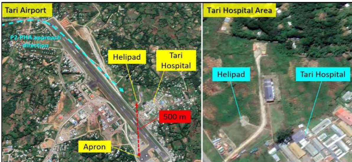
Figure 5: Helipad in reference to Tari Airport Apron
