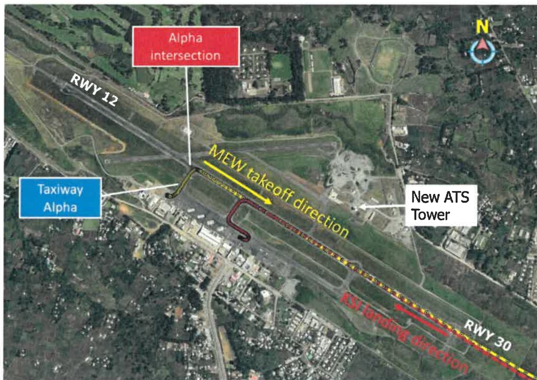
Figure 1: Mt. Hagen Airport runways and Control Tower
