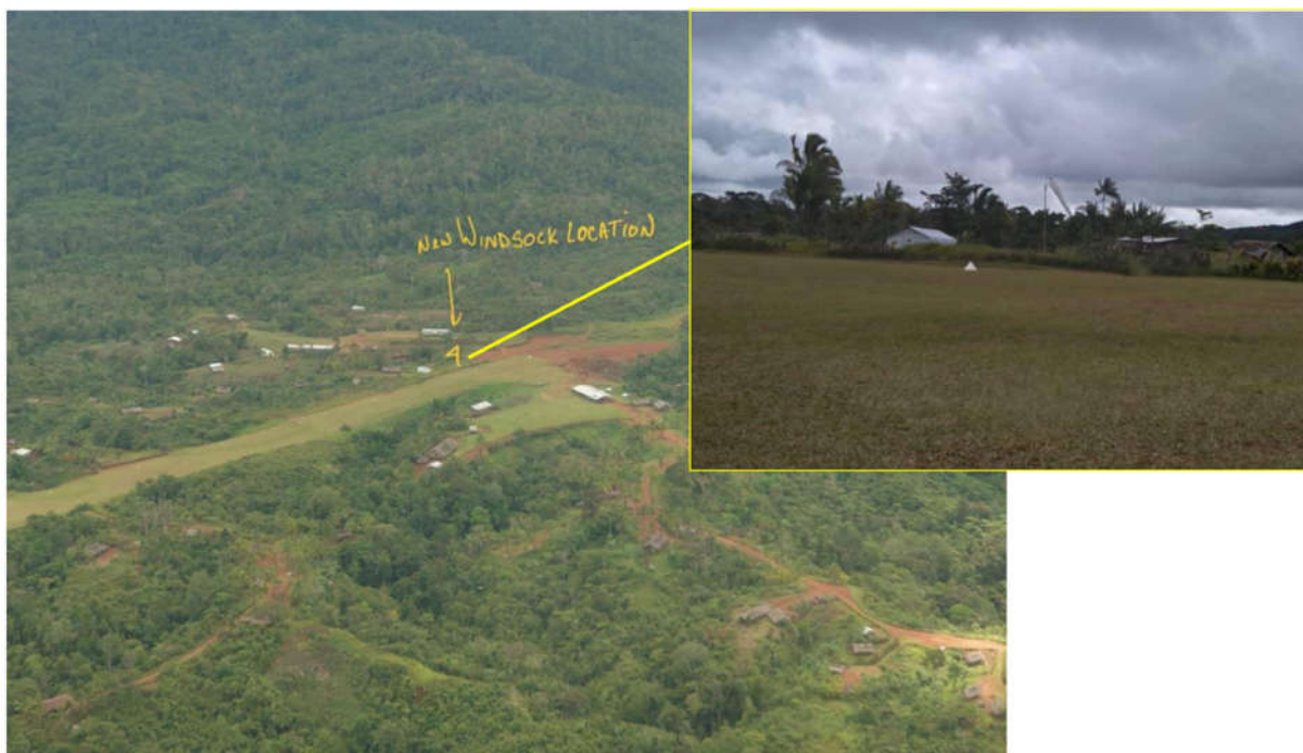
Figure 2: Dodomona Airstrip showing windsock near the take-off departure threshold
