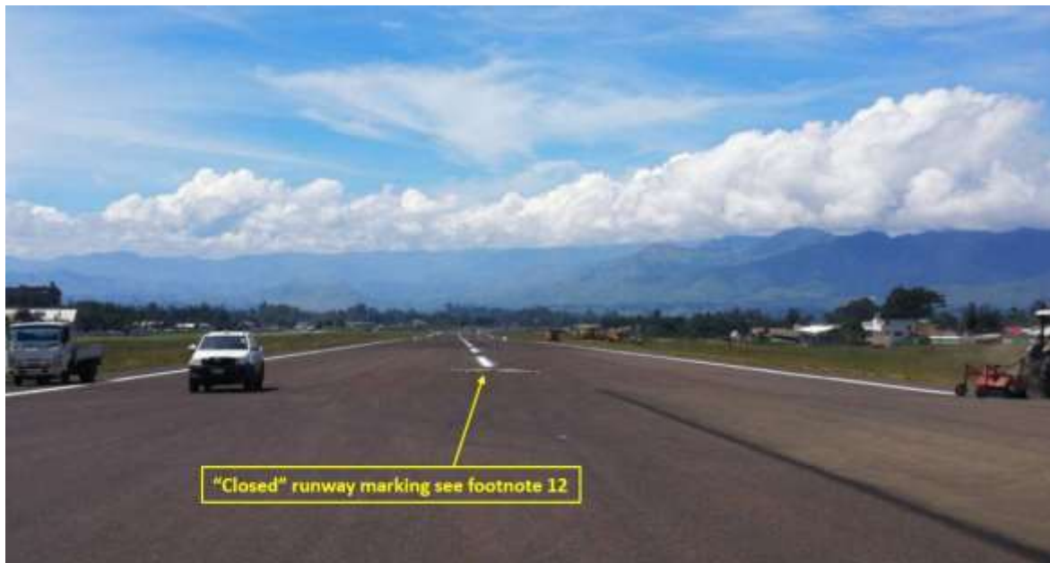
Figure 4 13 . Runway works in progress viewed from runway 17 Right.
