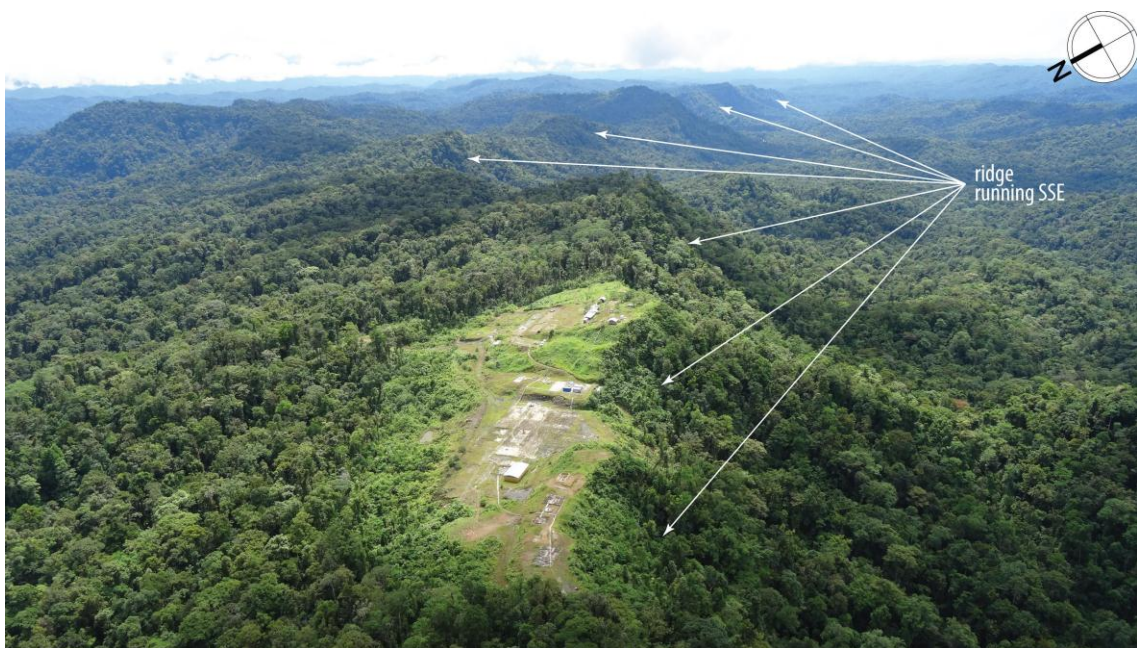
Figure 1: Triceratops 2 drill site, looking east south east along the ridge
