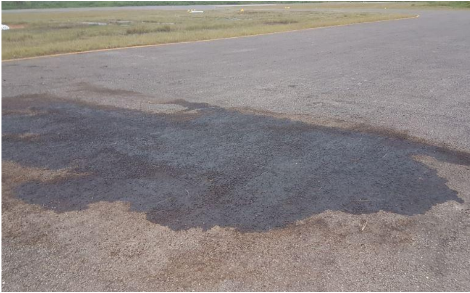
Figure 4: Fuel spill on the aerodrome apron
